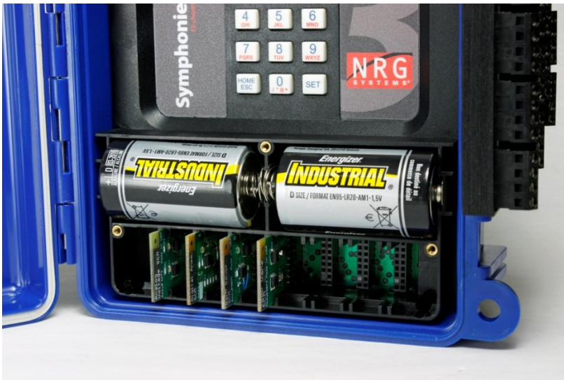
SCM cards installed under battery cover
